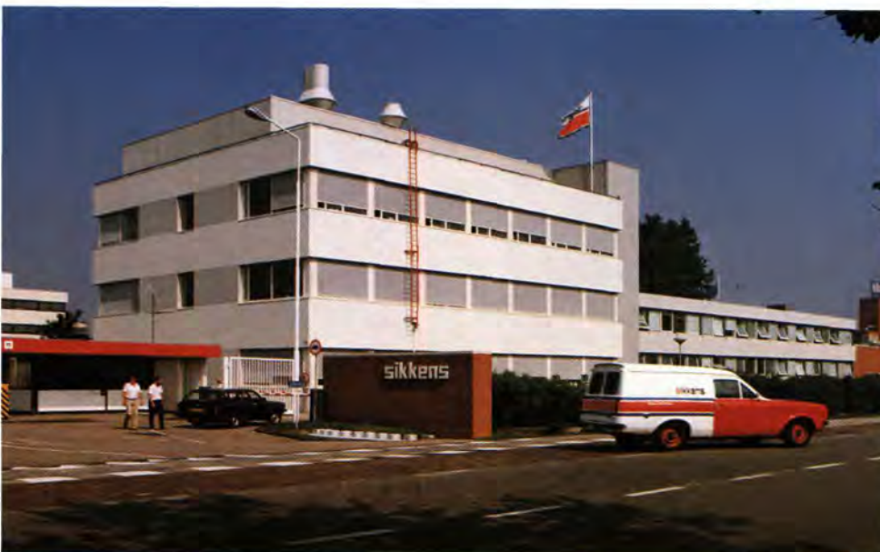
In the spring of 1984 a new wing of Sikkens' research building at Sassenheim was taken into use. It houses the polymer laboratory and the research laboratories for automotive and aircraft finishes.
