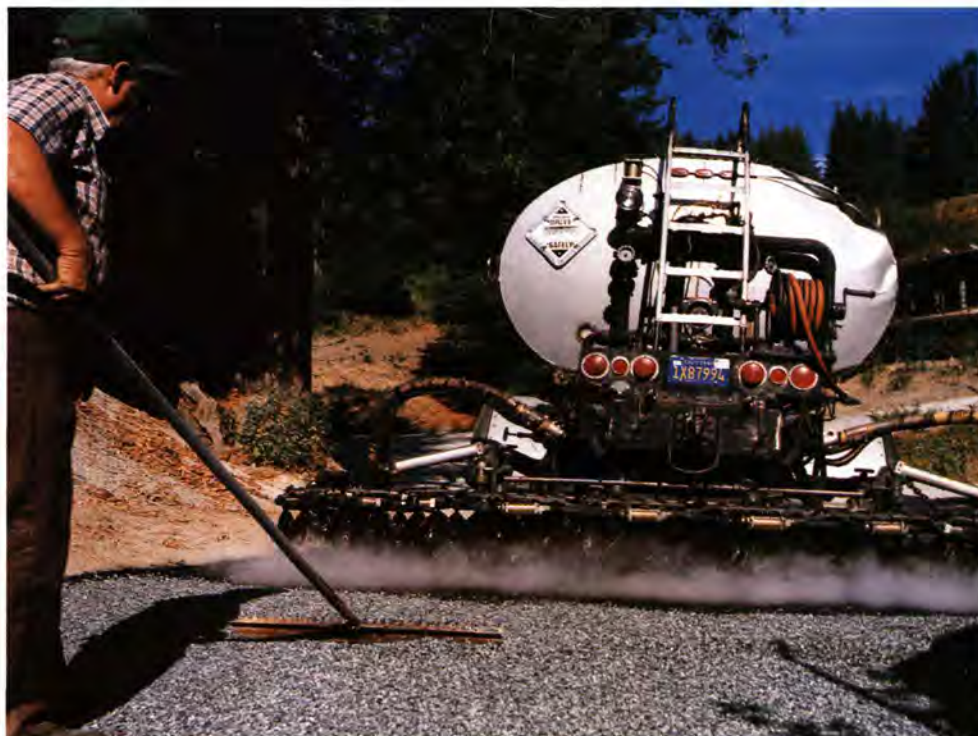
Akzo Chemie supplies road construction companies with Redicote® emulsifiers based on fatty amines. These bitumen additives ensure proper adhesion of the asphaltic layer to the rock or gravel subbase.
